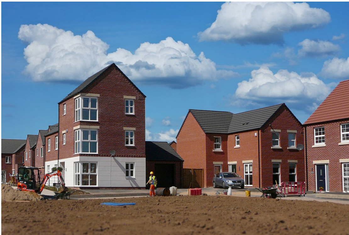
Photo 6: New housing under construction at The Edge, Clowne
