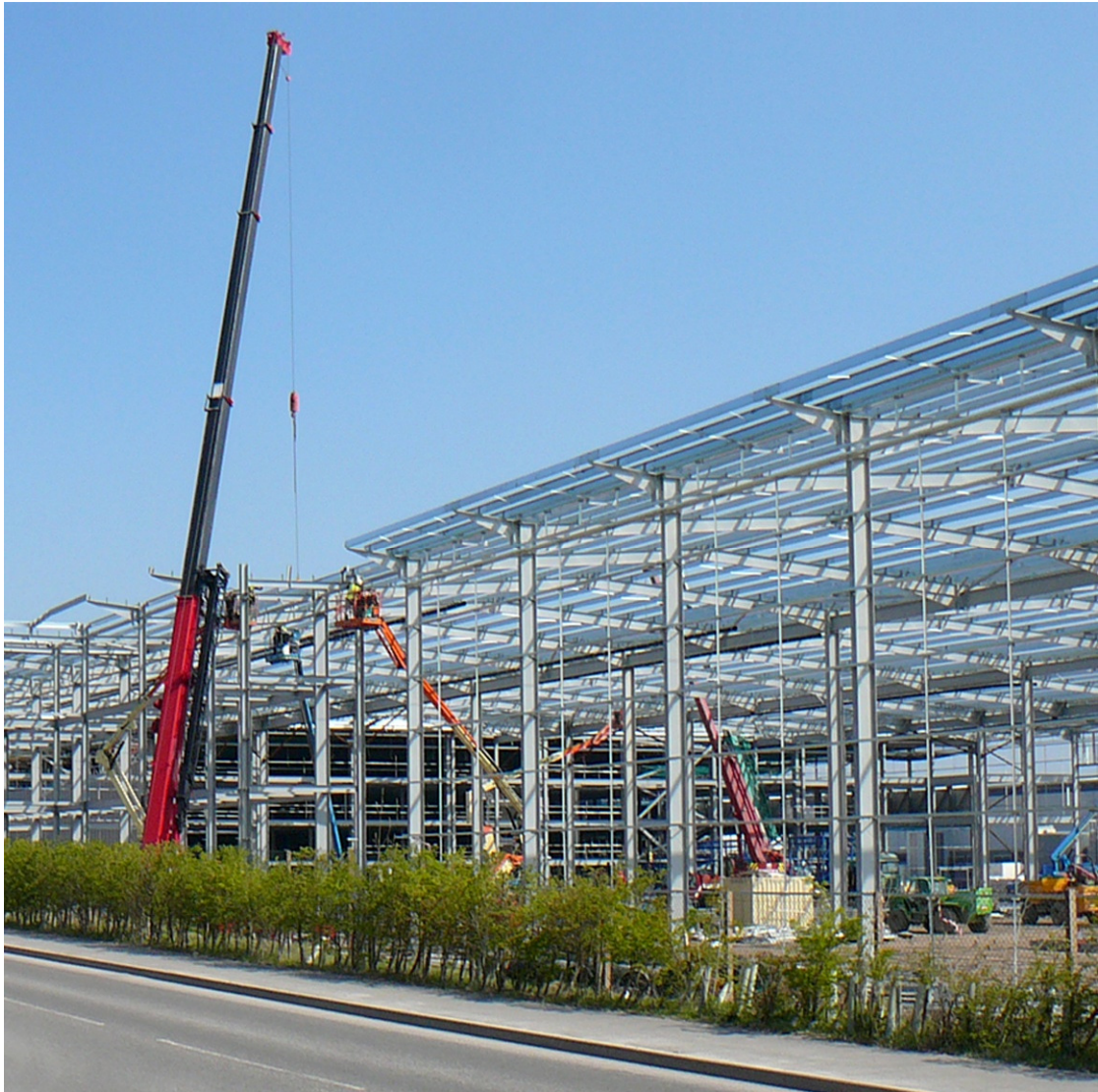
Photo 9: The Sports Direct distribution centre, under construction at Brook Park, Shirebrook
