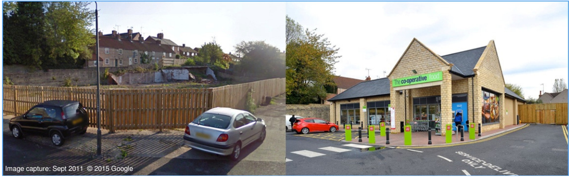
Photos 7 and 8: Before and after photographs of the new convenience store at Whitwell 6
